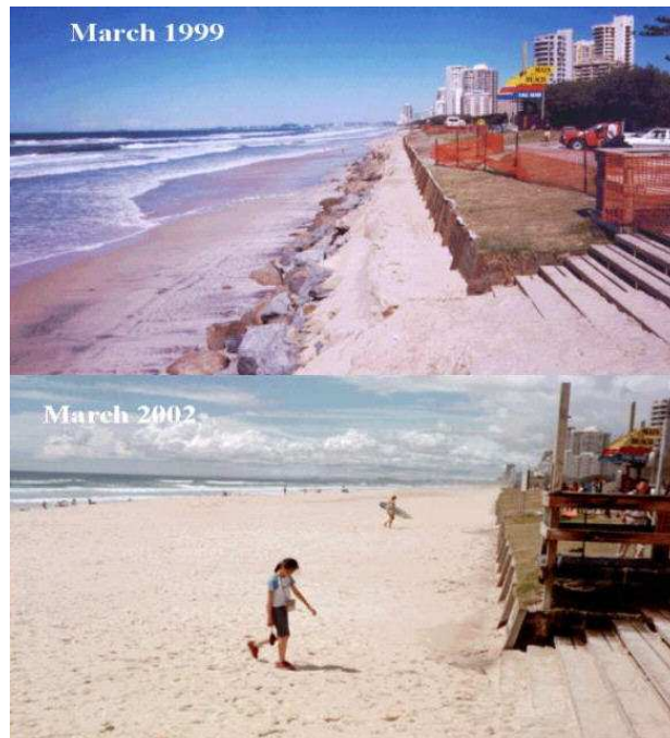
Before (top) and after (bottom) the construction of the Narrowneck multi-purpose reef on the Gold Coast, Australia.
