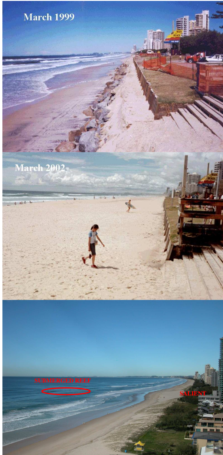
Figure 4. Coastal protection with the Narrowneck submerged reef. Top to Bottom: Before reef construction (construction commenced in August 1999); After reef construction; The view looking south showing the wide salient in the lee of the reef.
